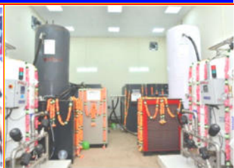
Pressure Swing Adsorption (PSA) Oxygen Plant at GB Pant Hospital
