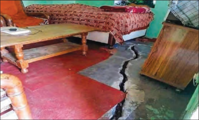
Wide crack on the floor of a house at Joshimath
